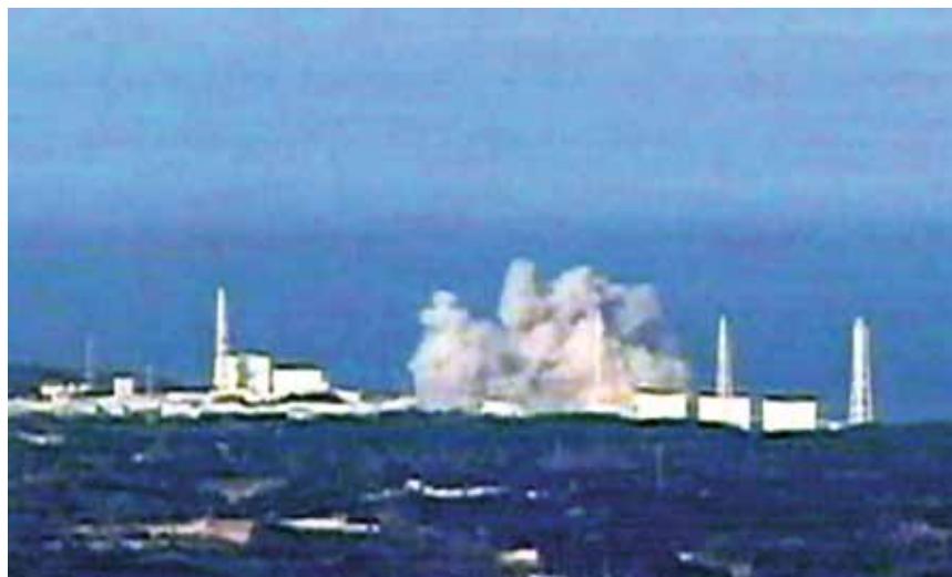
Figure 3: Hydrogen Explosion at Reactor Fuel Pool No. 4 March 15, 2011
