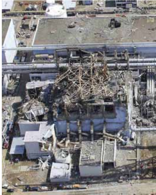
Figure 2: Reactor No. 3 Spent Fuel Pool Area
