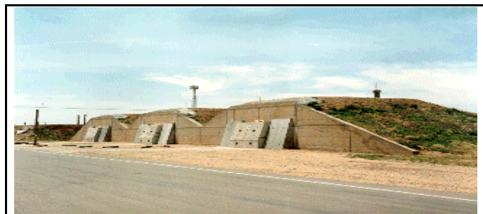
Figure 3-12. Zone 4 Bunkers at Pantex. Plutonium pits are literally stacked to the ceilings in these WWII and 1960’s vintage bunkers. All but a few of these facilities lack required humidity or temperature controls, and are unlikely to withstand an aircraft crash – a serious issue due to the proximity of Amarillo International Airport. Pantex has little space for additional pits.
