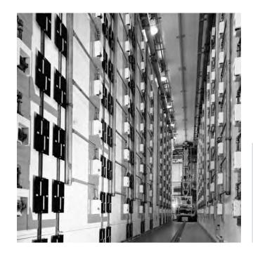
Figure 6 UK Sellafield Product and Residue Store, which became operational in 2011. Cans of plutonium are stored in separate lockers to protect against criticality accidents. *Source*: Sellafield Ltd.
